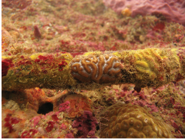
Figure 7.2 Delicate encrustations of coral and coralline algae on a fiber optic telecommunications cable. (Photograph courtesy of G. Rivera and S. Drew)
