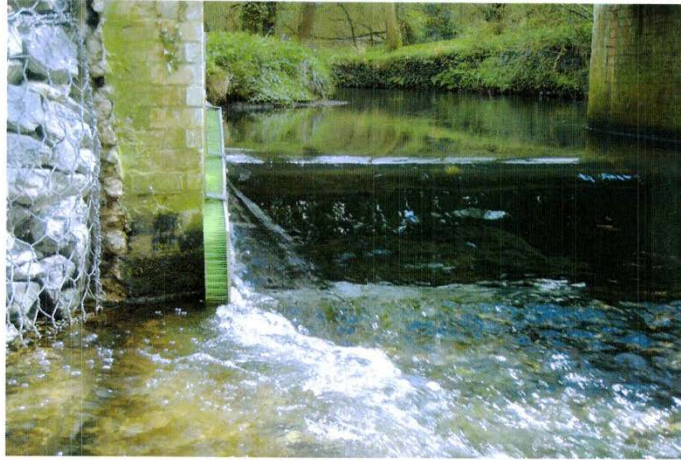
4.12 Downstream view of pass installation at Frog Mill, River Hamble (NGR: 5222 1491). Note the area of slack water on left for elver and eel to enter pass.
