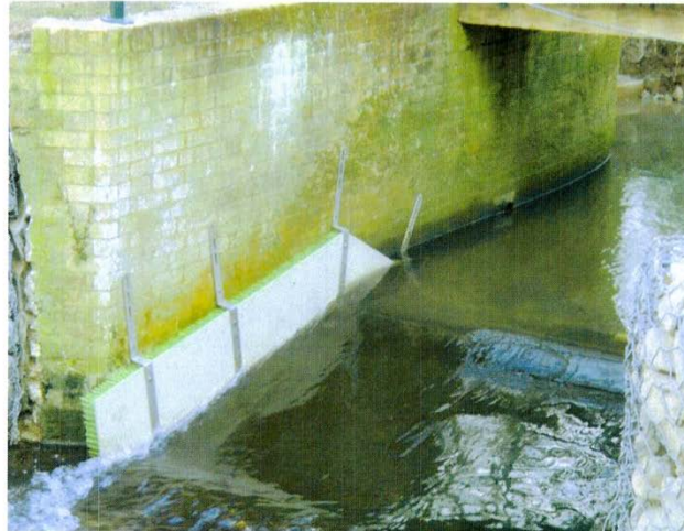
Figure 4.13: Installed pass, showing brackets and fixings
